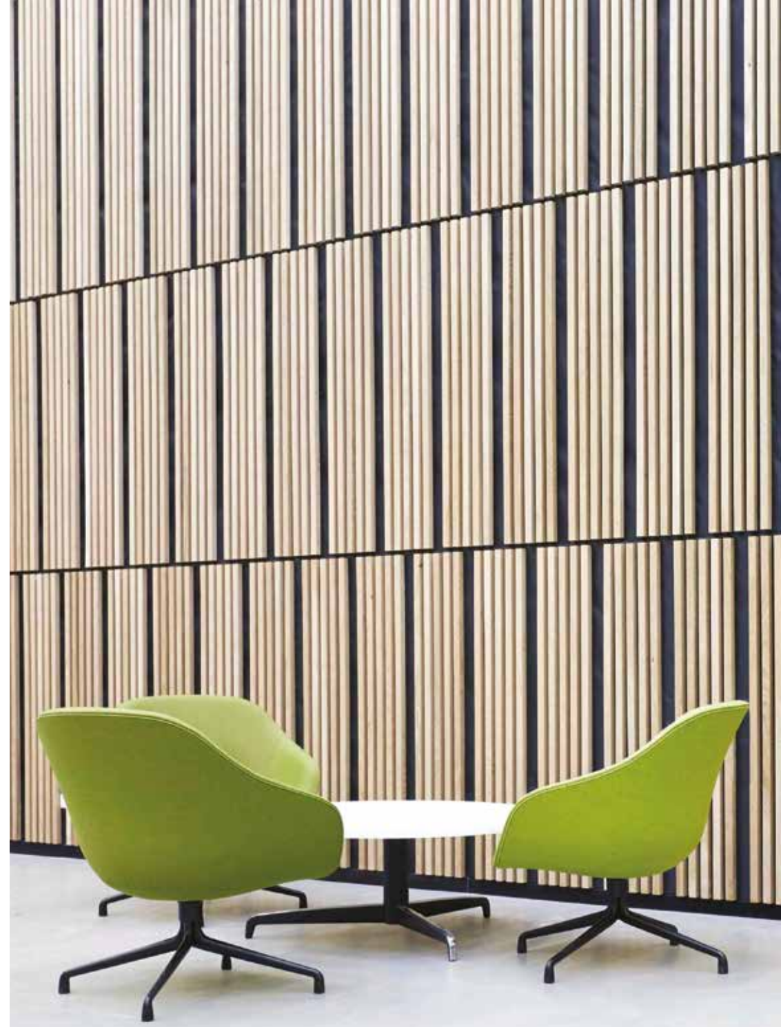
Interior sound-absorbing construction, flame retardant treated with C260.
